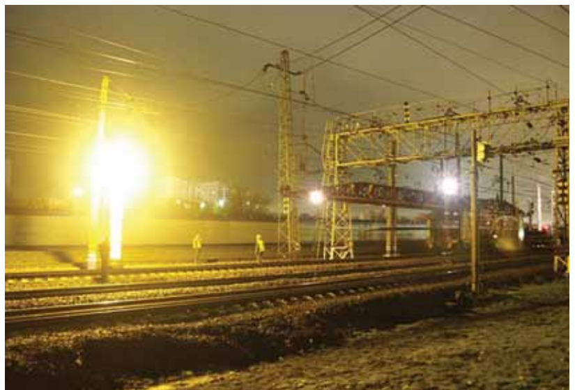
Night Track Works
